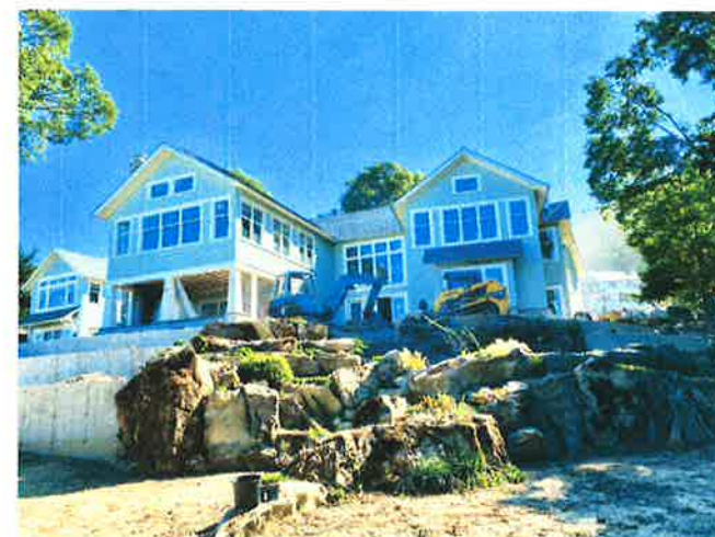
NORTH SIDE (REAR) OF 48 PROSPECT
