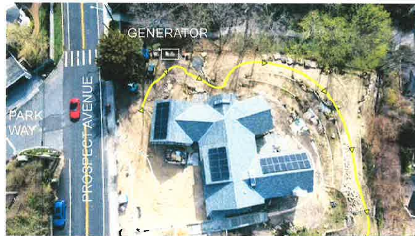
AERIAL VIEW OF 48 PROSPECT
